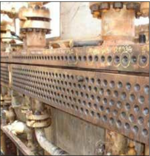
FinFan cooler before a maintenance
